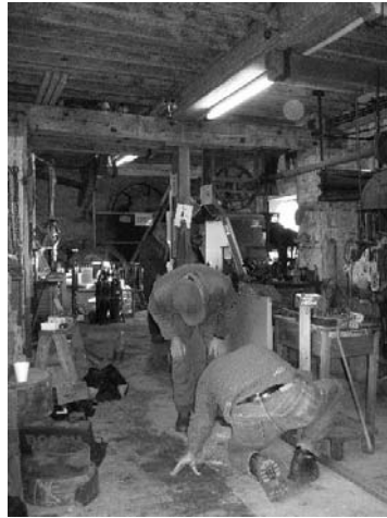
Ron and Chris Hayes work on the forge barrier
