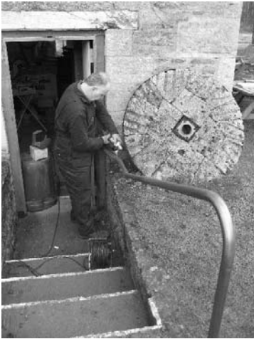
Nicholas preparing the new handrail for primer
